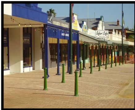
Main street after upgrade – removed kerbs for ease of access
